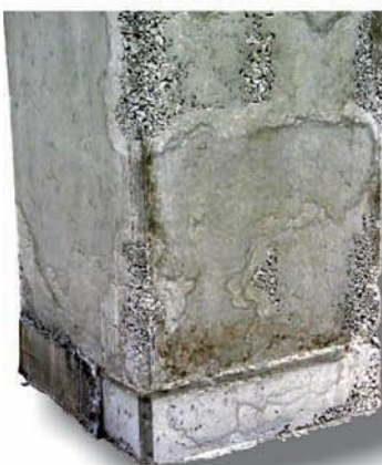
With high-cycle vibration in congested rebar
