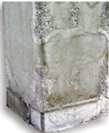
With high-cycle vibration in congested rebar
